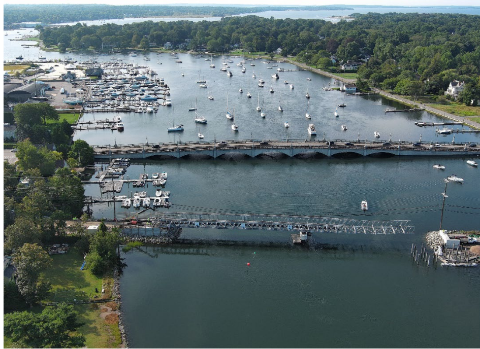
Warren Bike Path Bridge
