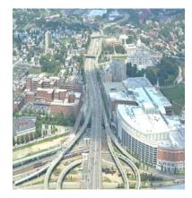
Interstate 95 North through the Providence Viaduct is the most congested highway in Rhode Island. This proposed project includes the replacement of the Northbound I-95 Providence Viaduct. Rebuilding the interchange and eliminating weaves will greatly reduce traffic congestion and significantly improve safety. Three of the six bridges in the interchange that will be replaced are structurally deficient, with five additional structures being rehabilitated.
