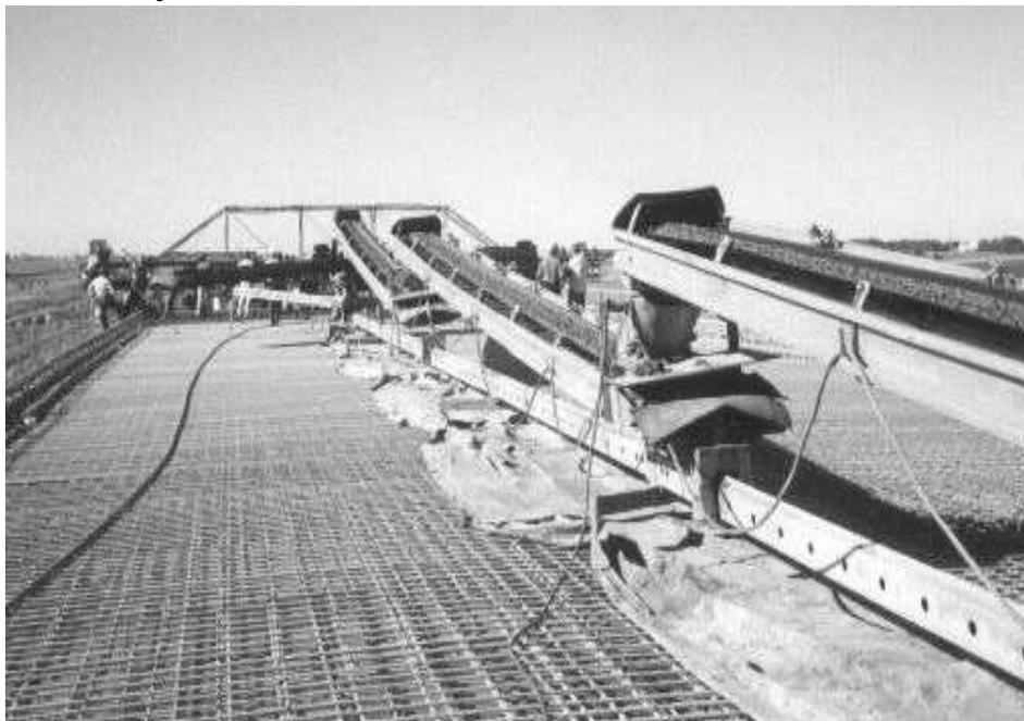
Typically, small amounts of loose mortar or concrete will spill from the sides of the conveyor belt, plastic or burlap should be placed directly underneath the conveyor
