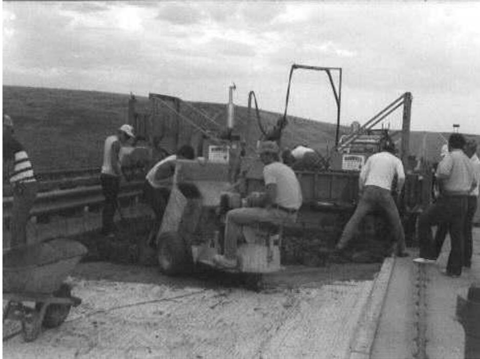
Hand buggies are two wheeled with rubber tires and have capacities of approximately 1/4 yard of concrete. They are pushed and dumped manually like a common wheelbarrow.
