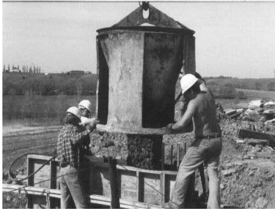
It is necessary to rest the bucket on a sheet of plywood or other material when it is being filled to prevent contamination with dirt. The concrete bucket should be filled by dropping concrete directly over the gate opening. Dropping concrete on the sloping sides of the bucket can cause segregation of the aggregate while filling.
