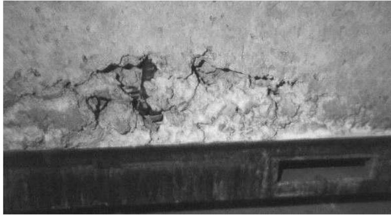
Small areas of honeycomb must be chipped out until solid concrete is exposed before being repaired. Several areas of honeycomb indicate poor procedures were used during placement. If severe enough the entire segment may require removal and replacement. Discuss this with your Project or Area Engineer before starting repairs.
