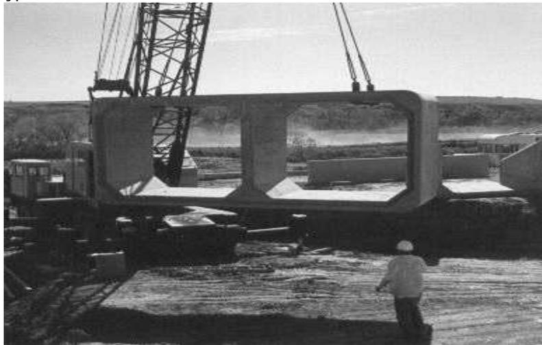
**Figure 1.13** Typical Cast-in-Place Box Culvert
