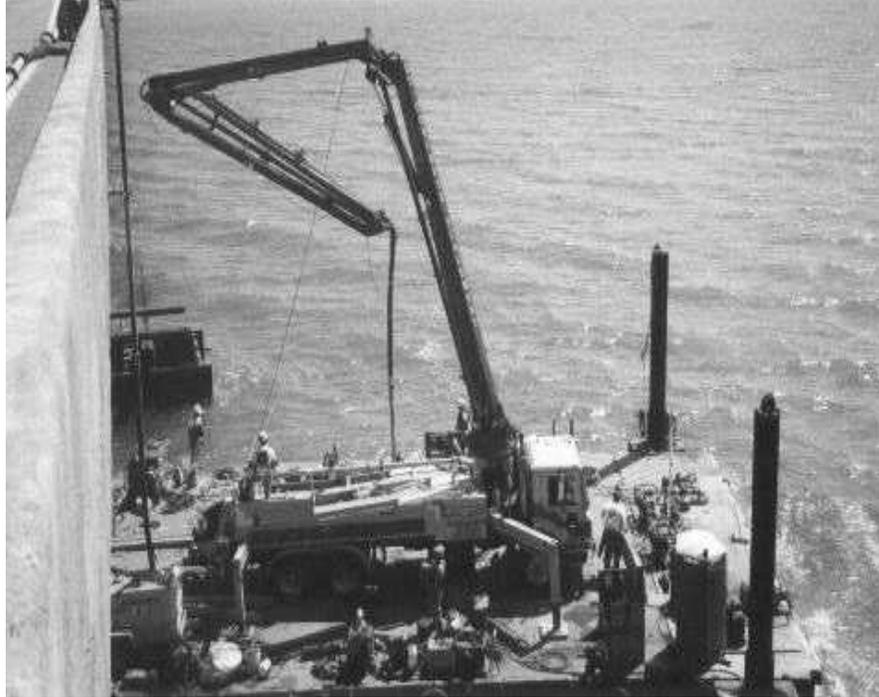
Typically pumps are initially flushed with a thin water/cement paste mixture to coat the lines. The grout lubricates and dampens the pipe walls, eliminating the loss of grout or water when the concrete is pumped. Do not allow this grout to be used for the concrete - waste it!
