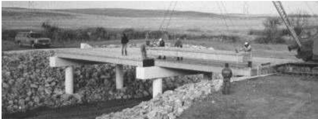
**Figure 1.10** Bulb Tee Bridge
