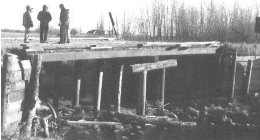
**Figure 1.9** Precast Double Tee Bridge
