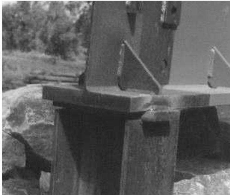
These are generally the only welds made in the field because most high stress connections are bolted. Welds made in high stress areas must meet rigid requirements, including tests for weld subsurface quality as determined by Magnetic Particle Testing, Ultrasonic Testing, or X-rays. Welding in high stress areas, unless specified in the plans, is not allowed without prior approval of the Bridge Construction Engineer.
