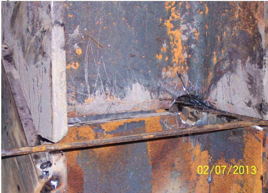
When set-up procedures don't provide the bearing needed, a pile splice is required. Be sure the contractor has the materials to make splices before driving pile.
