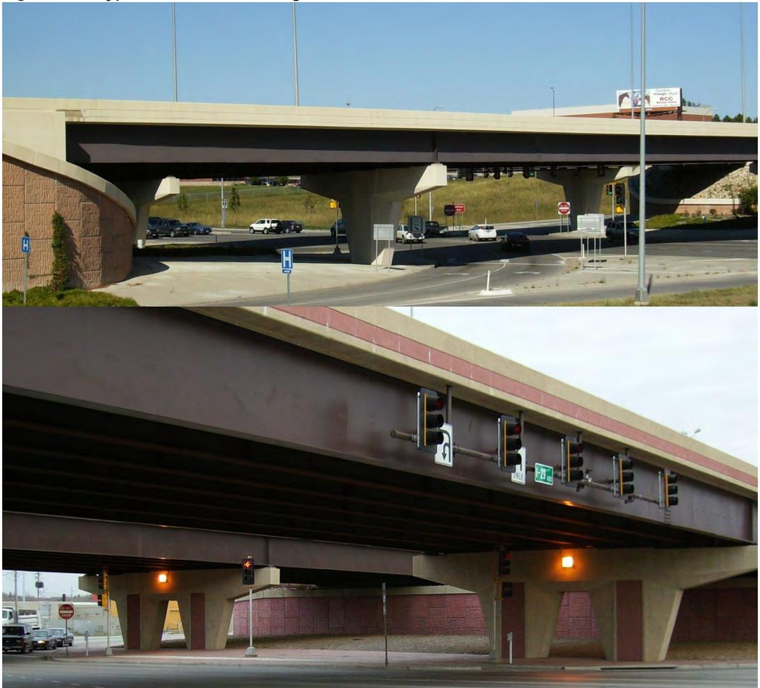
**Figure 1.3** Typical Prestressed Girder Bridge
