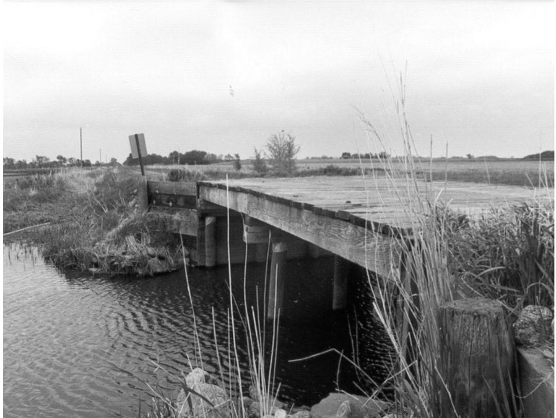
One of the most common applications for timber on new bridges is that of timber abutments or timber bents. Figure 15.4 is a typical plan sheet showing a timber abutment for a precast channel bridge. This chapter will cover applications of permanent timber construction beyond the typical timber piling. Timber piling is covered in extensive detail in 'Chapter 4 - Piling'.
