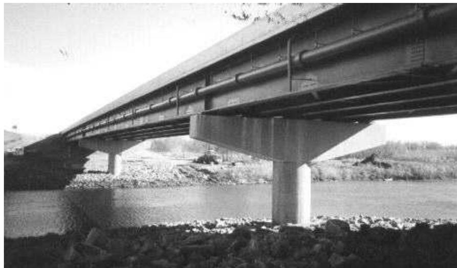
**Figure 1.17** Typical Multi-Column Bent
