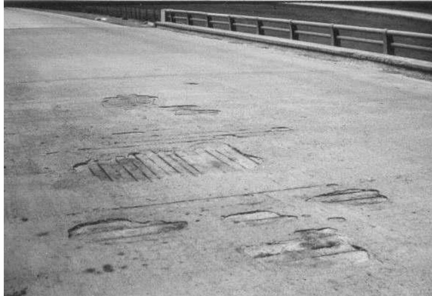
The designers assume that the proper cover will be maintained, although at times this may be impossible. Therefore, accept the work as meeting the cover requirements if the following construction tolerances are maintained: The cover should be maintained within  $\pm 1/4$  inch of the plan specified amount. Check the cover distance with a measuring tape, and if the cover that is needed is not being maintained, have the Contractor place additional devices to properly support the bars.
