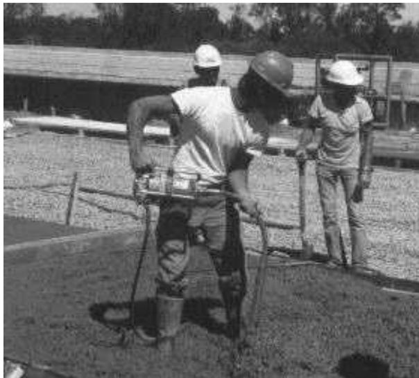
**Rule of Thumb** Let the vibrator penetrate the concrete to the desired depth under its own weight. Pull it out of the concrete at the same rate as it entered.
