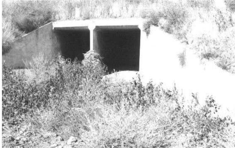
**Figure 1.12** Typical Precast box section
