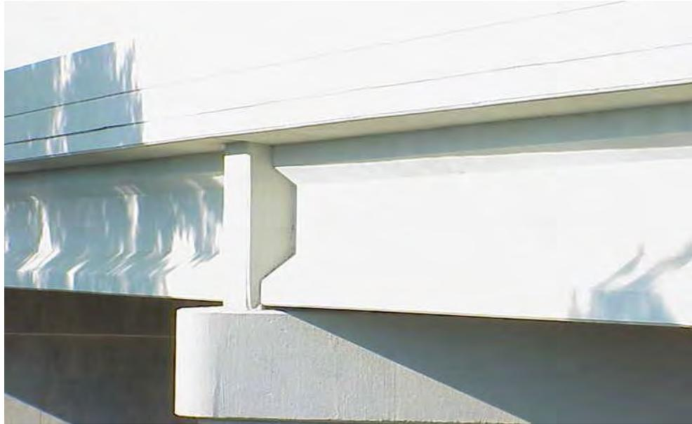
**Figure 13.2** Steel Girder Bridge
