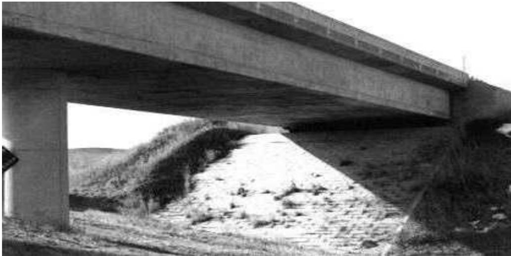
**Figure 1.7** Concrete Rigid frame
