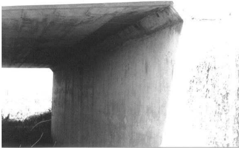
Concrete in forms will generally have a smooth surface when the forms are removed. When the surfaces are not in view of the traveling public, the only finishing required is what is necessary to fill holes left by ties or honeycombing. Honeycombing is similar to a rock pocket. It occurs when concrete is not vibrated thoroughly, resulting in rock not surrounded with fines and grout.
