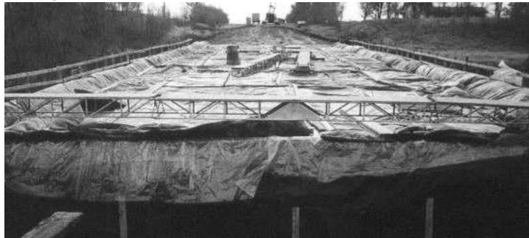
Heated enclosures keep the workmen out of bad weather. Check to make sure they are reasonably airtight so cold air does not reach the concrete. You should also see that the enclosure is big enough to maintain at least one foot of clearance between it and the forms. This is needed so the warm air is free to circulate around the unit.
