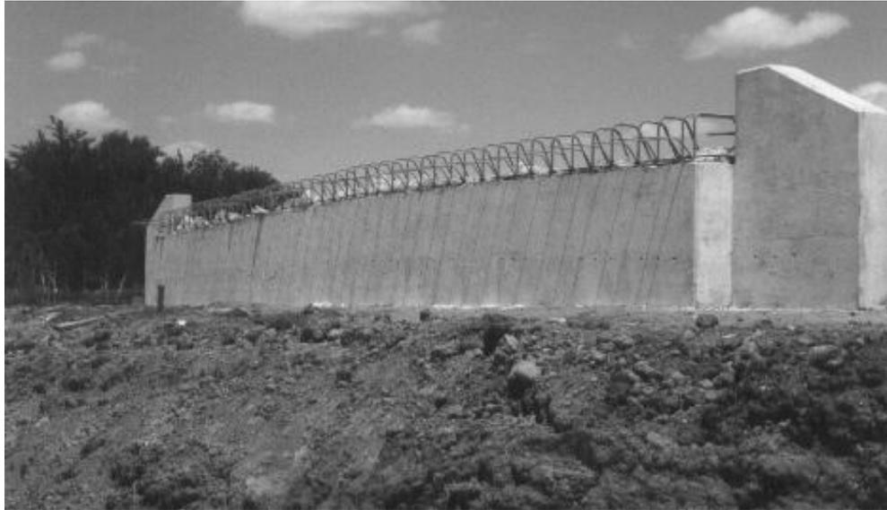
The bents or piers are the interior foundation units that support the superstructure loads. Several types of bents or piers exist, ranging from large single columns with cantilevered caps on each side (typically called hammerhead piers) to multiple columns with a concrete cap (acting as a beam) to even a full bridge width concrete wall (commonly called a pier wall). The following are examples of common bridge bents or piers.
