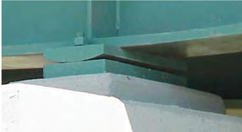
The anchor bolts on the sliding plate type or the fixed device can be tightened. The sliding plate has a self lubricating plate below the flange that allows movement. The fixed device remains stationary.
