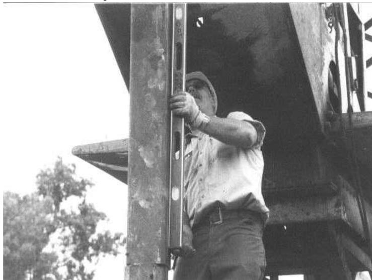
**Figure 4.4** Measuring from Offset to Kelly Bar
