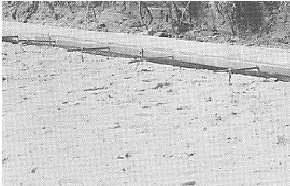
**Figure 3.28** Keyway strip in slab.
