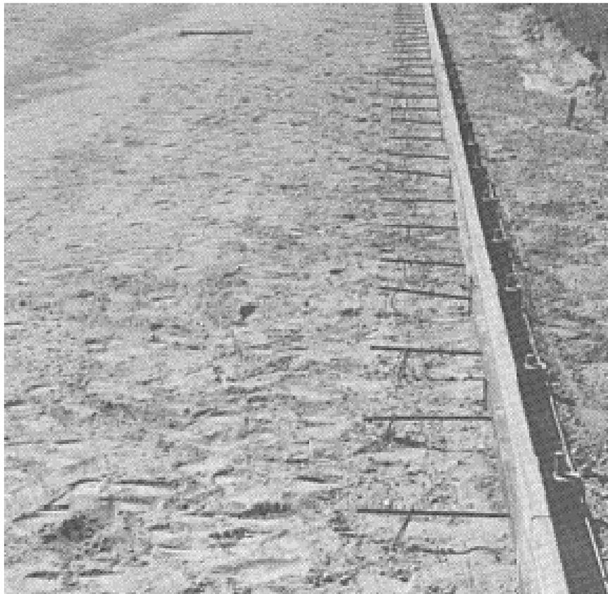
**Figure 3.9** Top curb is uneven from poorly set forms.
