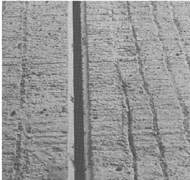
**Figure 7.8** Beveled edge transverse contraction joint after the pavement surface has been ground.
