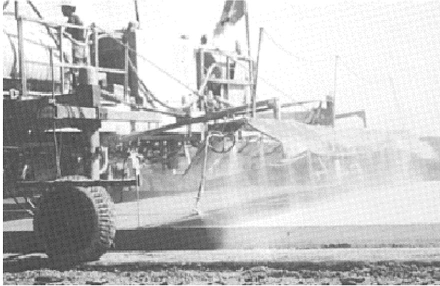
**Figure 6.15** Curing machine. Note the 1) wind skirt on the back, and 2) curing compound tank and agitating machine at the left on top of the curing machine bridge.
