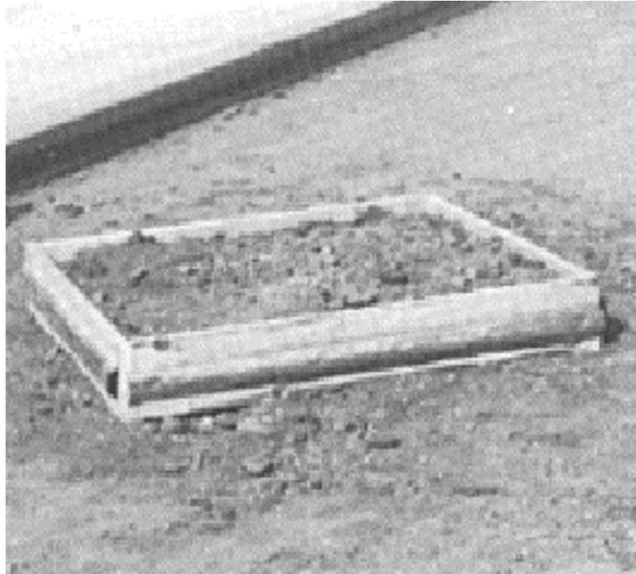
**Figure 3.12** Drop inlet box in place before paving.
