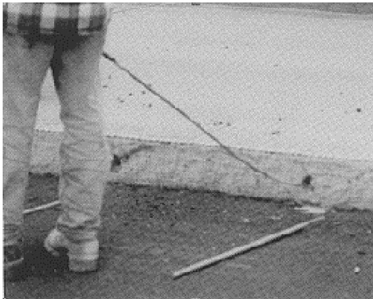
**Figure 3.23** Crew placing tie bars
