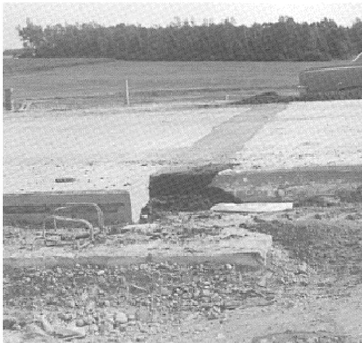
**Figure 7.19** Strip Seal Expansion Joint
