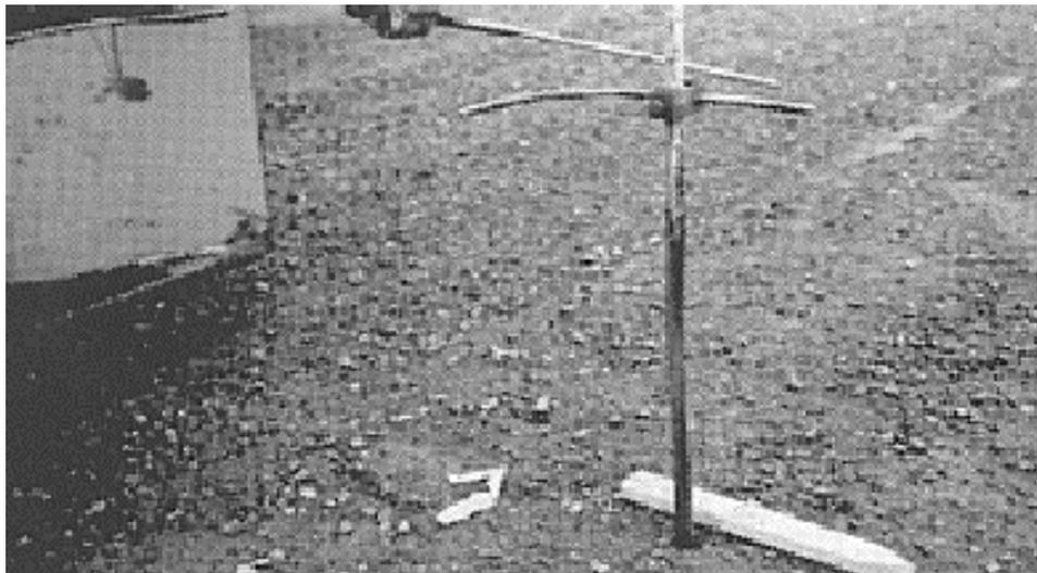
**Figure 7.2** Paint extending toward centerline from orange ribbon nailed to ground marks the intended joint location.
