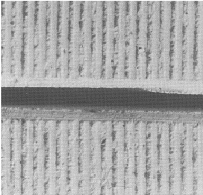
**Figure 7.9** Sawed joint. Note the disturbance of the curing compound covering the slab.
