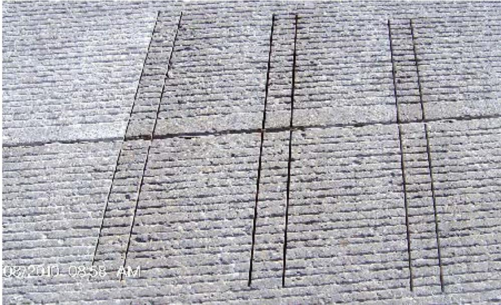
**Figure 9.7** Dowel bar retrofit installation
