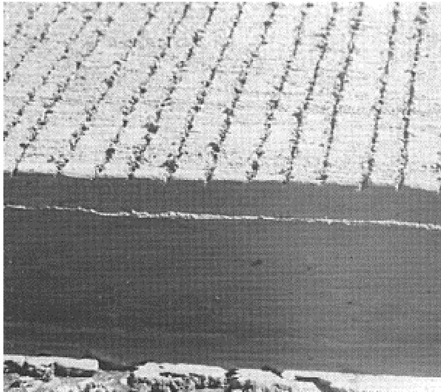
**Figure 6.7** Tining machine in operation. The wooden slats, (strips of light metal or belting material may be used) to cover joint areas to be sawed.
