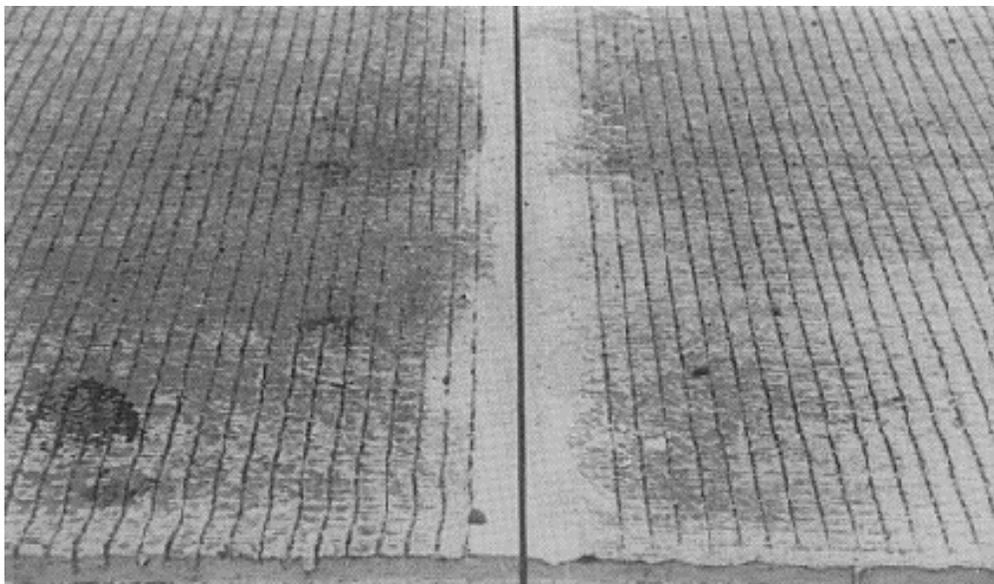
**Figure 7.10** Sawed joint and resulting cracking of slab.
