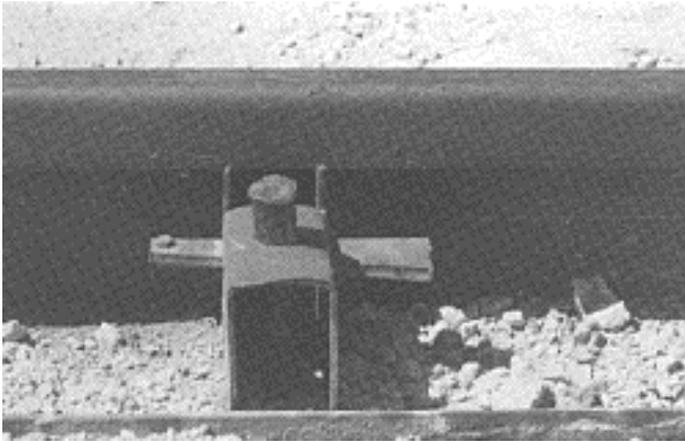
**Figure 3.4** The arrow points to the form sliding end piece for locking together adjoining forms.
