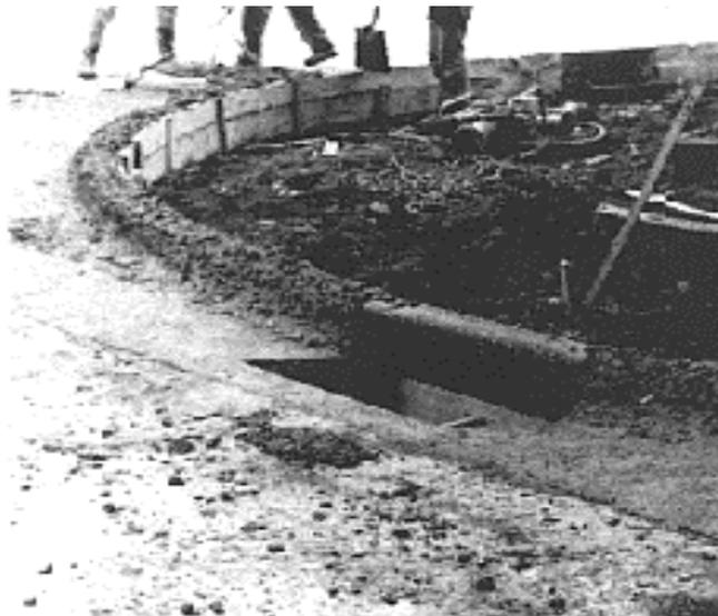
**Figure 8.4** Hand edging and finishing curb and gutter.
