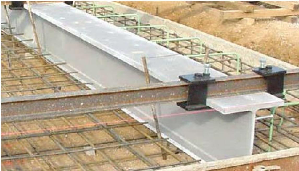
**Figure 4.16** Setting pavement terminal.
