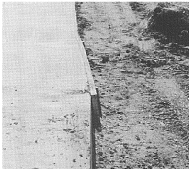
**Figure 7.23** Finishing the start of concrete placement at the header. Note the damage being done to the curing compound. This should be re-sprayed.
