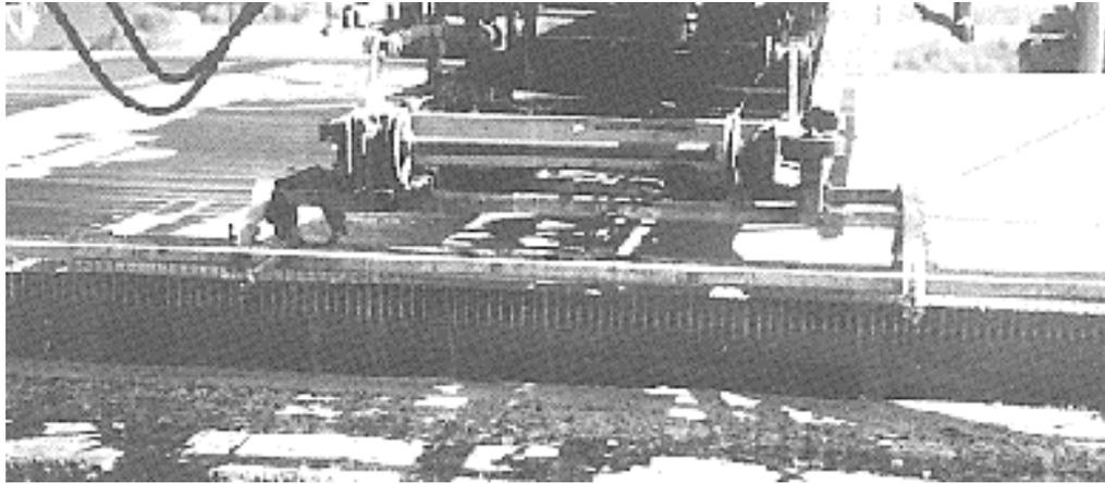
**Figure 6.9** Tines picking up aggregate indicates poor consolidation.
