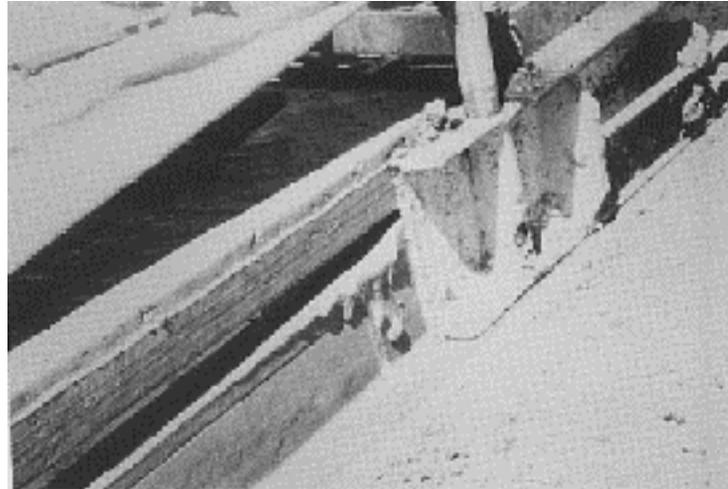
**Figure 3.30** Keyway formed on the outside of the pavement.
