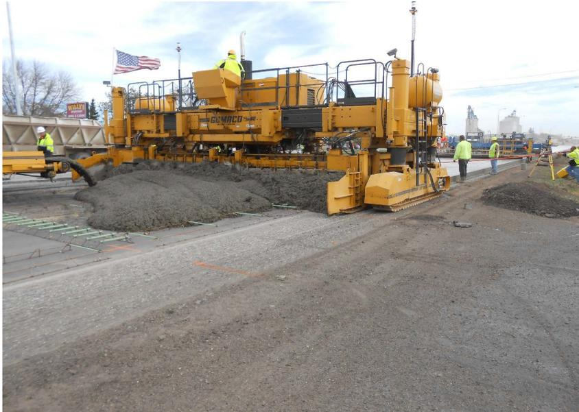
**Figure 5.6** Stringless (Slipform) Paver is guided by Universal Total Station System.
