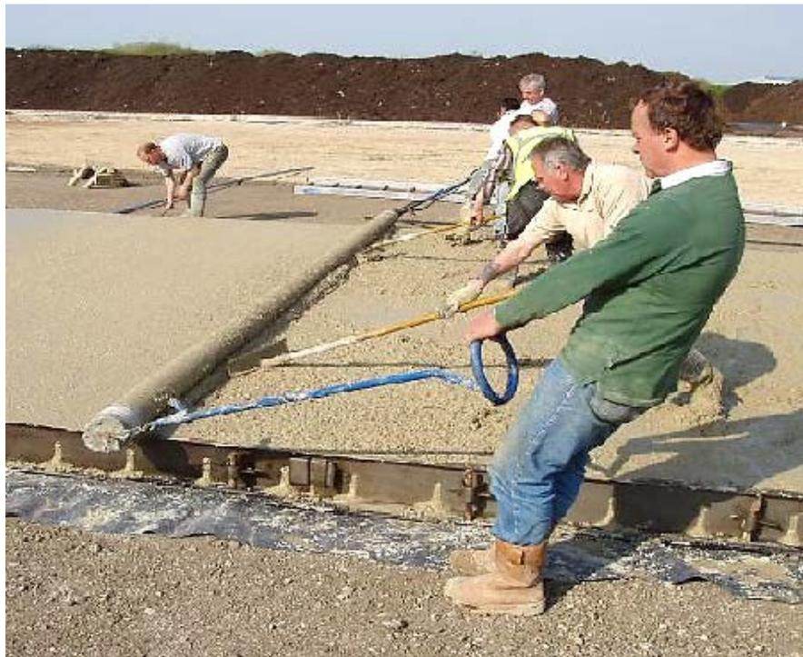
**Figure 5.24** Picture of a Truss Screenshot which is used for small formed placements. These screeds normally have cable and a winch that moves the screed forward.
