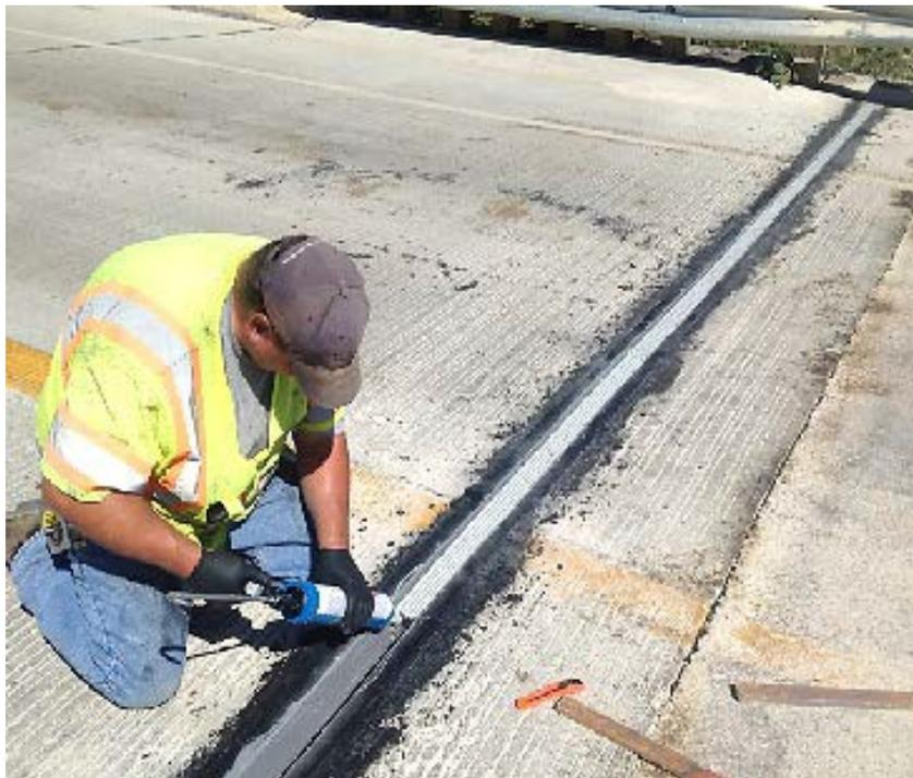
**Figure 7.17** Membrane Seal
