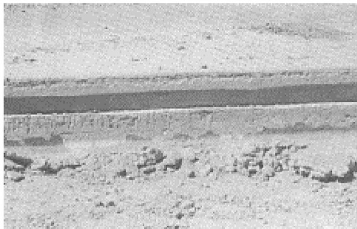
Some slipform pavers feed a metal keyway into the front of the paver (Figure 3.29). This continuous metal keyway keeps the top edge from slumping down after the slipform process. The keyway is held at the proper height through the paver by a small lip on the inside surface of the side forms of the paver. Tie bars can even be installed during this process.
