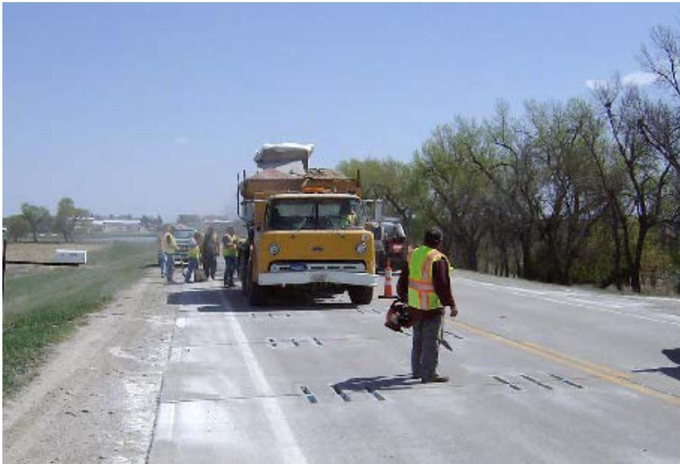
**Figure 9.8** Curing of dowel bar retrofit
