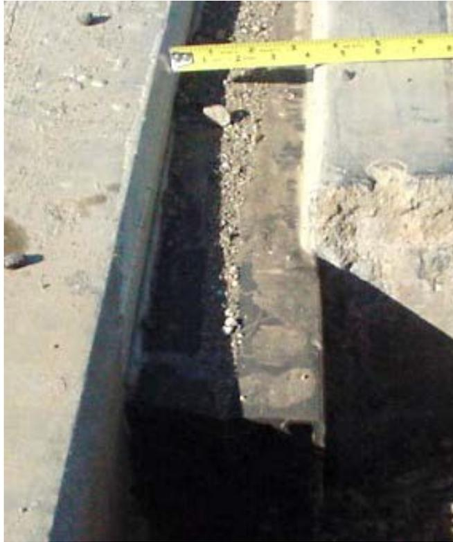
**Figure 7.16** Membrane Seal Installation
