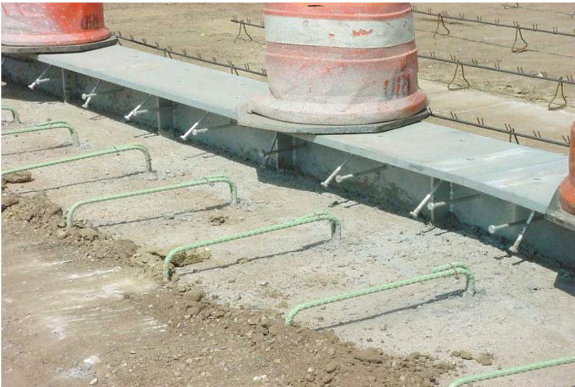
**Figure 4.18** Nonreinforced side completed and asphalt bondbreaker placed.
