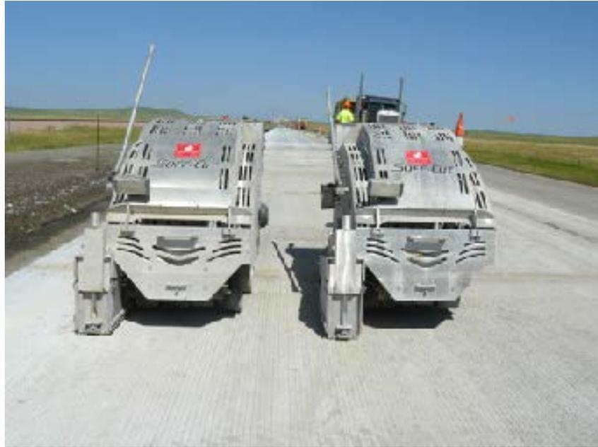
**Figure 7.5** Concrete saw.
