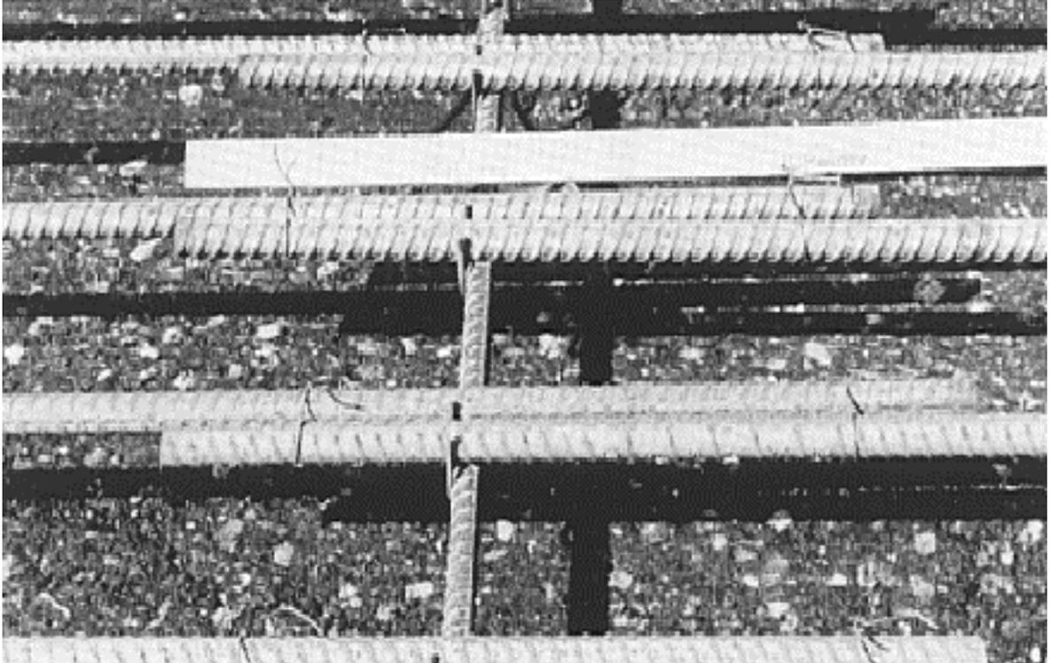
**Figure 4.8** Checking steel placement spacing.
